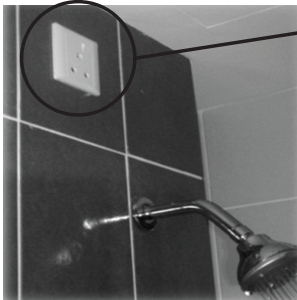
Figure 1 - Example of a socket placed in bathrooms, to be replaced with a Splash Proof Connector.
